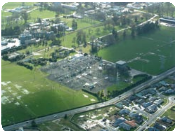
The Substation reporting point, located inside the City Sector of the Hamilton Control Zone.
