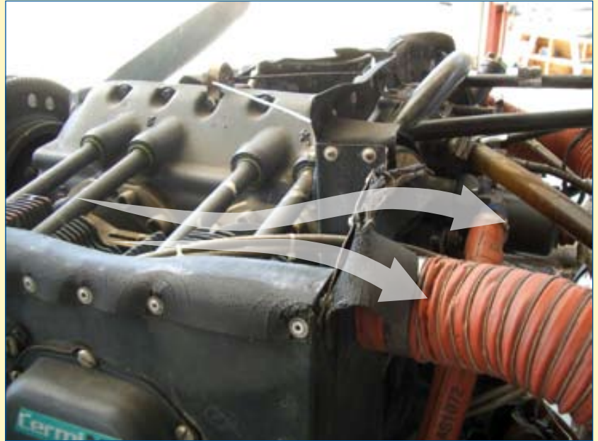
Old, torn and perished baffle seals lead to loss of cold air pressure resulting in engine overheating.
